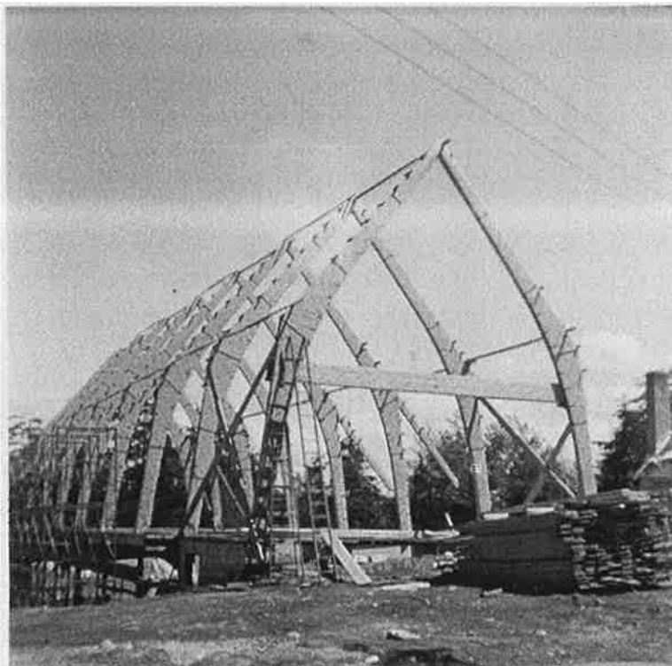
Arches for the new Sanctuary
